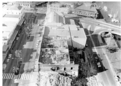
The demolition has begun. 1978
